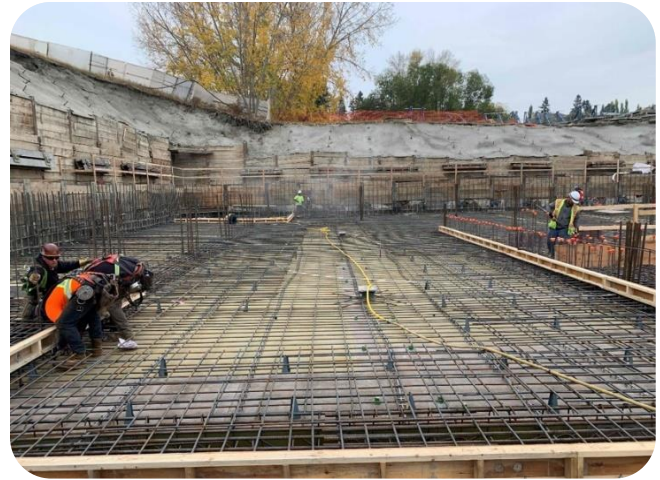
Main Floor slab rebar install
