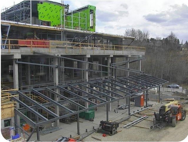
Southeast corner – concrete pour and structure steel installation completed
