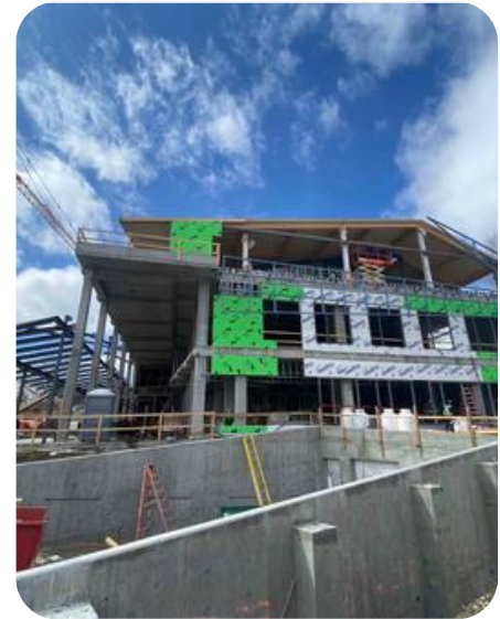
Ramp walls with east elevation
