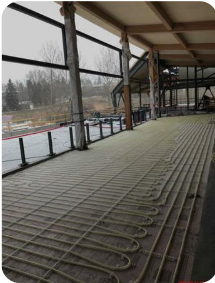
Level 3 in slab heating lines in place
