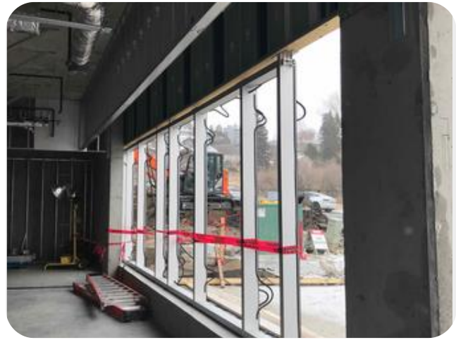
East wall glazing frame install underway
