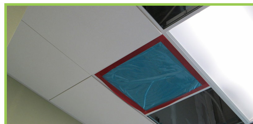
HVAC Equipment Protection from debris and dust during construction
