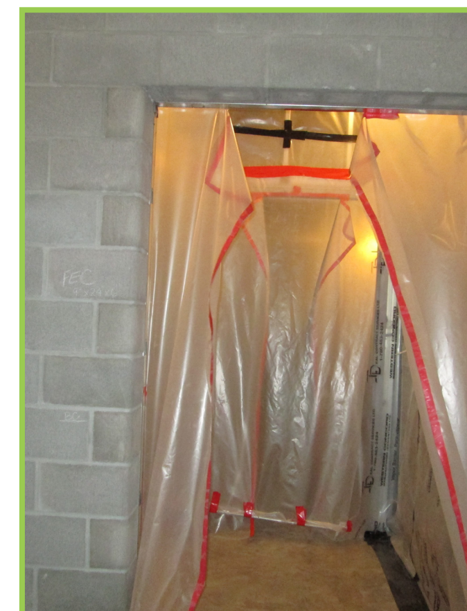
Barrier installed to isolate construction areas from clean or occupied areas.
