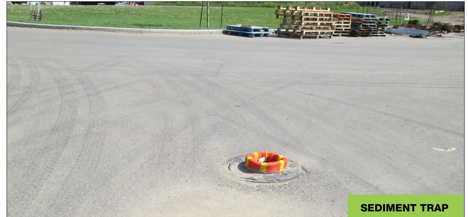
HAUL ROAD CLEANING
